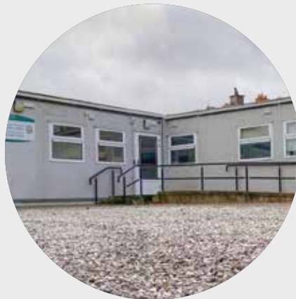
Gaol Road Campus Kilkenny R95 Y6PH
